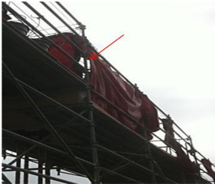
Fig. 2: Close-up of containment structure with arrow at gap.
